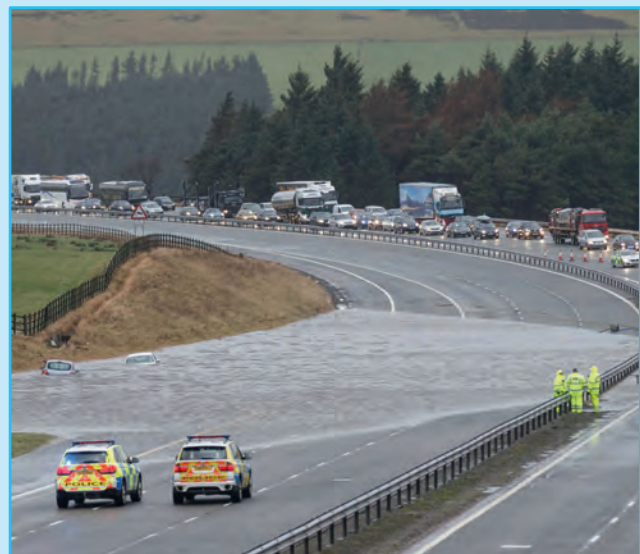
Flooding at M74 near Abington, South Lanarkshire after Storm Frank
